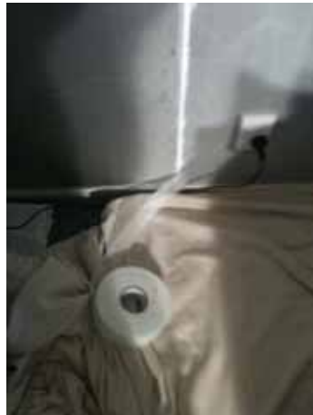
Start by sealing joins using Fibermesh tape
