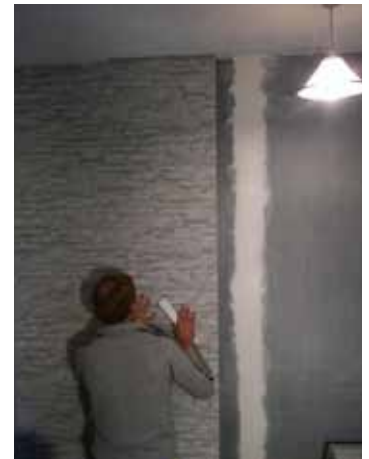
Once the wall has been 'sized' and allowed to dry wallpaper can be applied.
