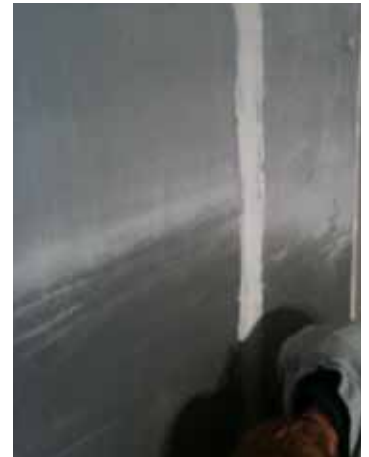
Example of FIBERMESH tape and plaster applied along the vertical joins
