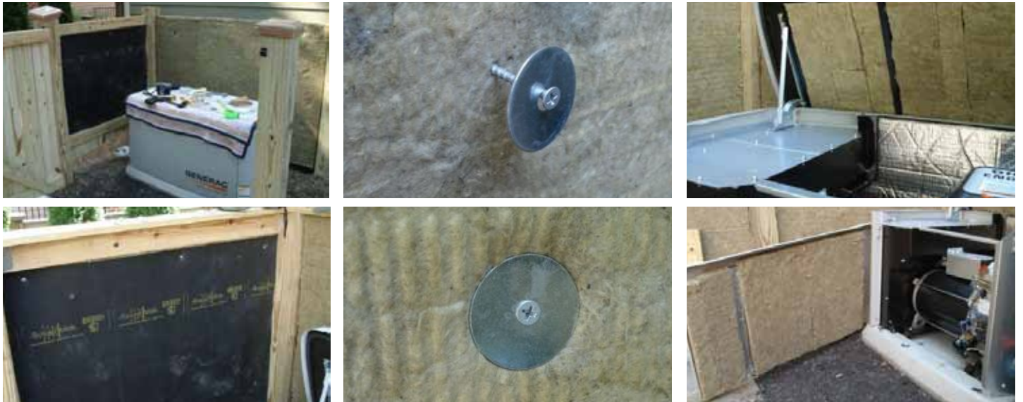
After Acoustiblok® application
